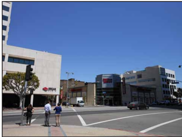
View 24: View from the southwest corner of Masselin Avenue looking north at the two-story commercial retail (Office Depot) building.
