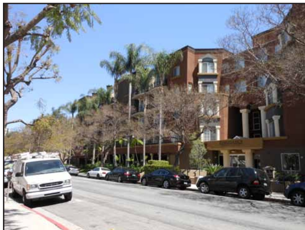
View 27: View of the five-story Renaissance Apartment Homes building.
