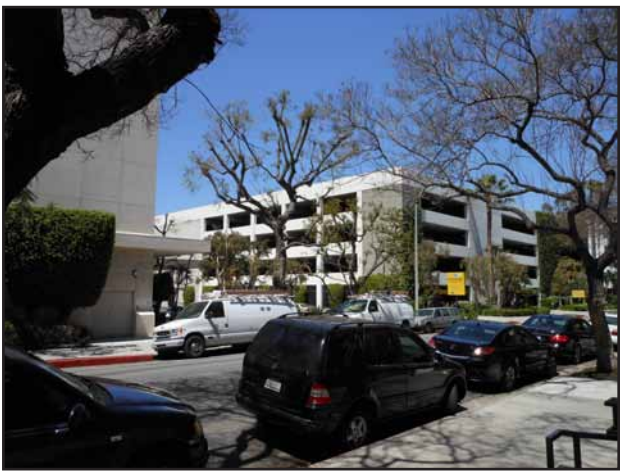
View 23: View from Masselin Avenue looking north at the project site's five-story parking structure and entry driveways.
