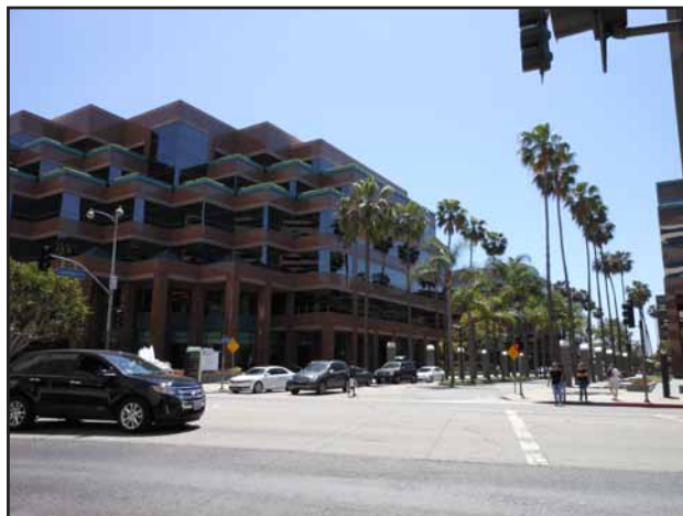
View 36: View from in front of the Museum Square complex, looking south towards the Wilshire Courtyard complex, down the center internal access road.
