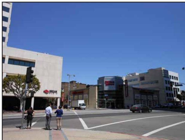
View 24: View from the southwest corner of Masselin Avenue looking north at the two-story commercial retail (Office Depot) building.
