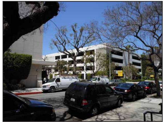
View 23: View from Masselin Avenue looking north at the project site's five-story parking structure and entry driveways.
