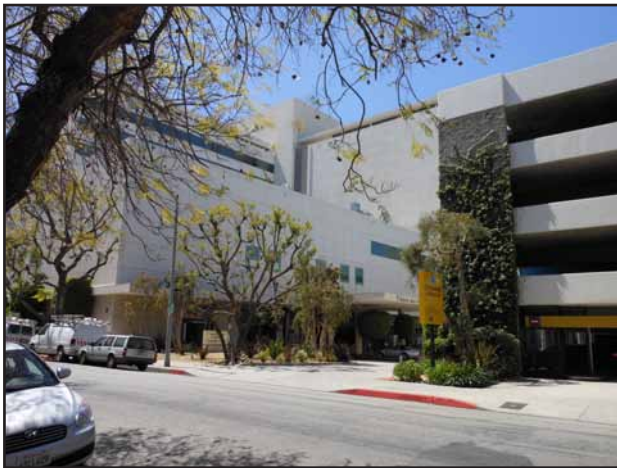
View 21: View from Masselin Avenue looking south at the Project Site's five-story parking structure and entry driveways, with the Museum Square 11-story office building.
