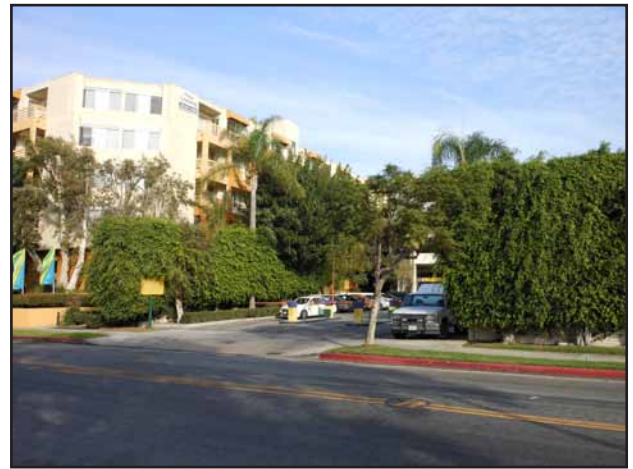
View 17: View from Curson Avenue looking east that the project site – northern driveway entrance.
